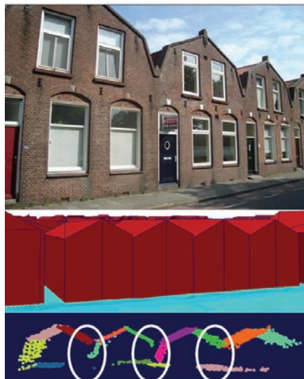
Figure 5-6 Gambrel roof types (top) are often modelled as gable roofs (middle), caused by missing laser segments at the lower roof faces of the gambrel roof (bottom) because of occlusion by the higher roofs.
