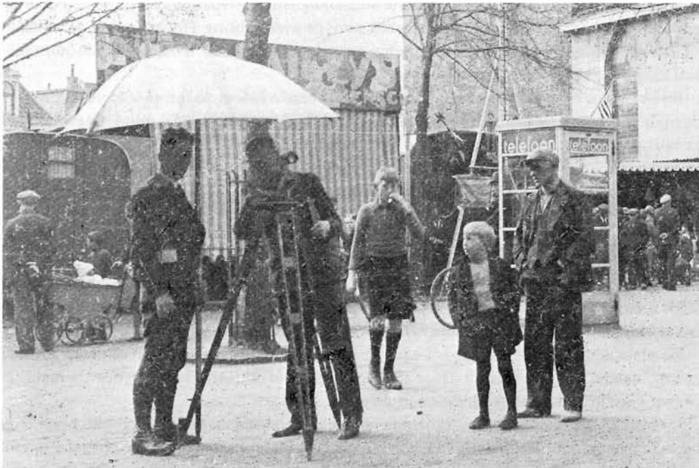
Fig. 25 Waterpassing door de stad. Levelling through a built-up area.
